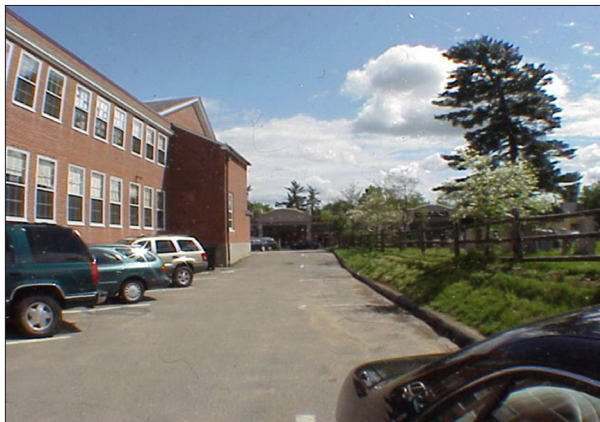
◀ ACCESS TO CEMETERY BEFORE CONSTRUCTION
