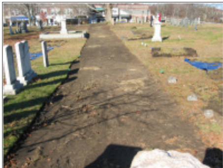
▲ PATH EXCAVATION: SURFACE REMOVED
